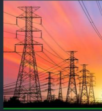
Grid Modernization Program Services
