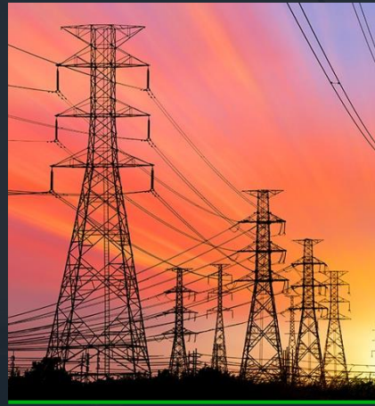
Grid Modernization Program Services
